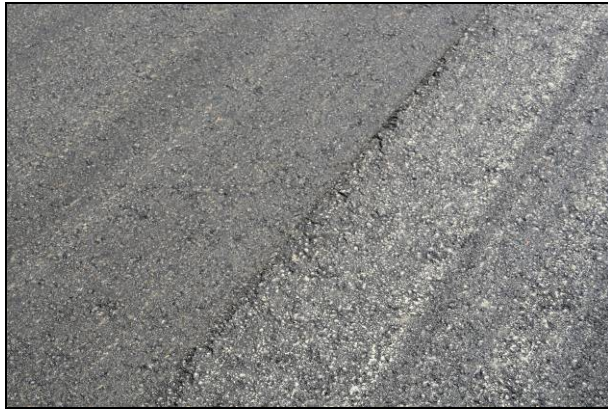
Figure 2.39: Sasobit: Surface after final rolling.
