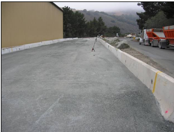
Figure 2.11: Completed base-course showing tightly bound surface.
