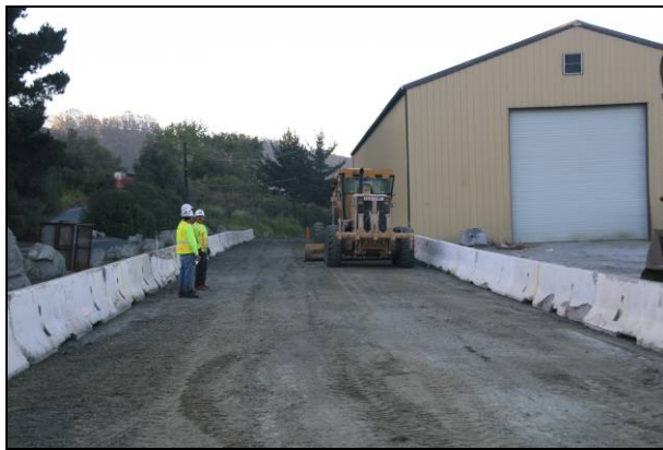
Figure 2.7: K-rail placement and subgrade/subbase preparation.
