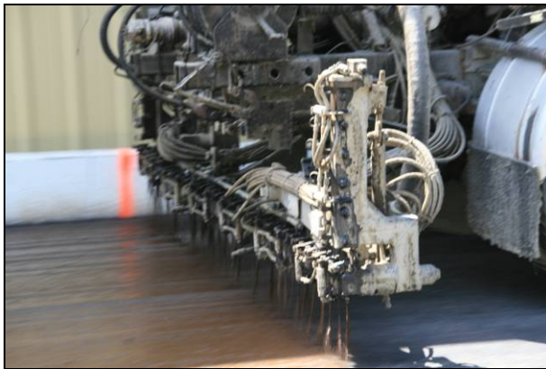
Figure 2.41: Tack coat application (Control).
