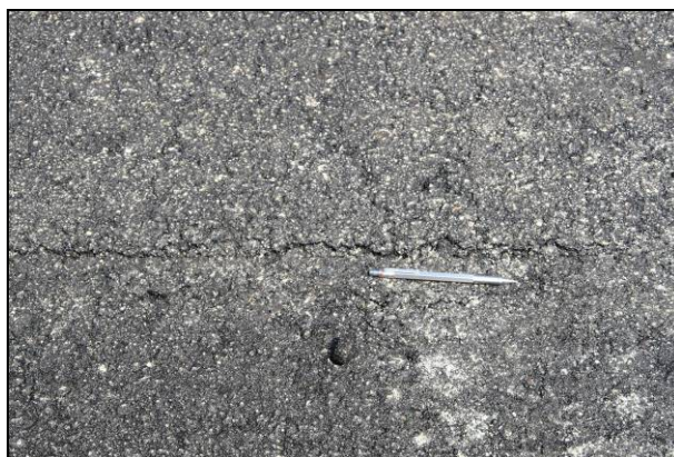
Figure 2.37: Sasobit: Shearing during breakdown rolling.
