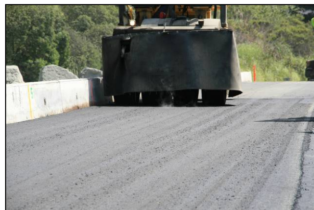
Figure 2.38: Sasobit: Pick up during rubber-tire rolling.
