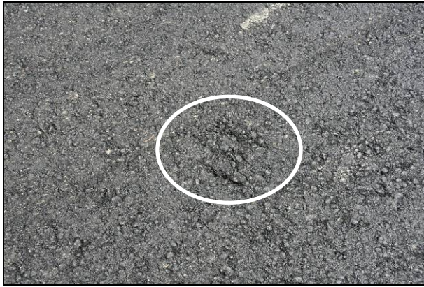
Figure 2.35: Evotherm: Shear after rubber-tired roller.
