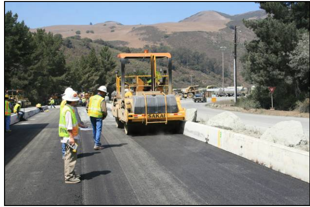
Figure 2.36: Evotherm: Surface after final rolling.
