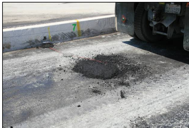
Figure 2.44: Strain gauge covered with mix.
