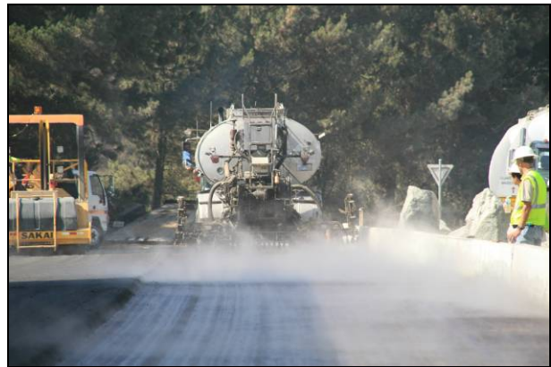
Figure 2.42: Tack coat application (Sasobit).
