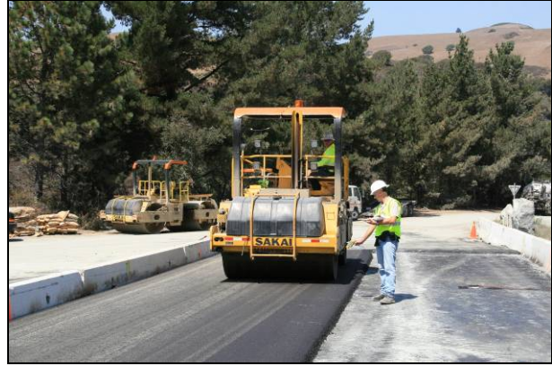
Figure 2.32: Advera: Surface after final rolling.
